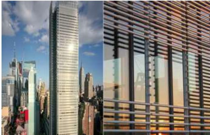
Fig. 10: New York Times Building Fig 11: Detail of ceramic shading elements
